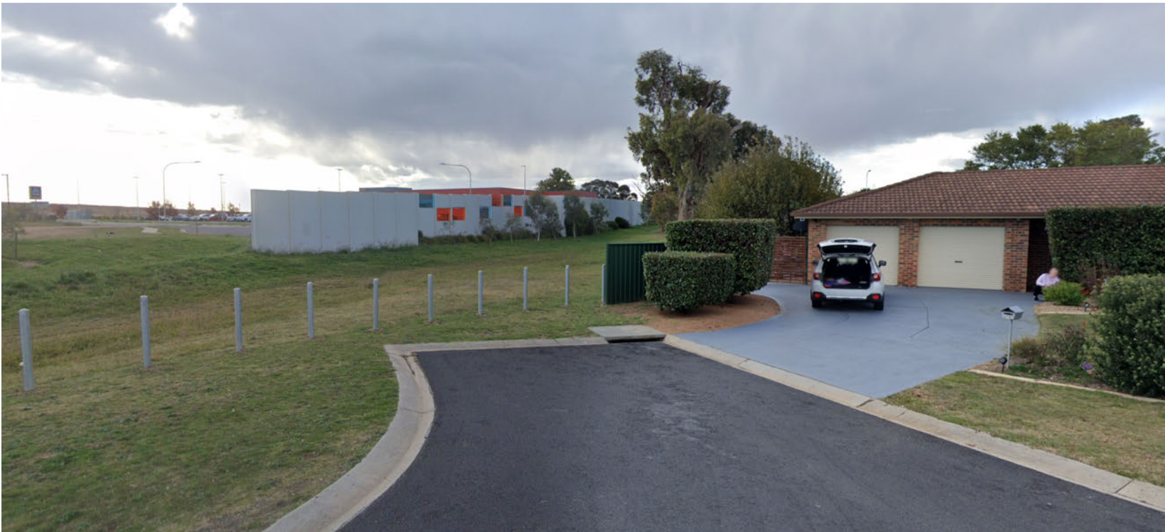
VIEW OF EXISTING 3.5m ACOUSTIC WALL FROM FRANKLIN Ct
