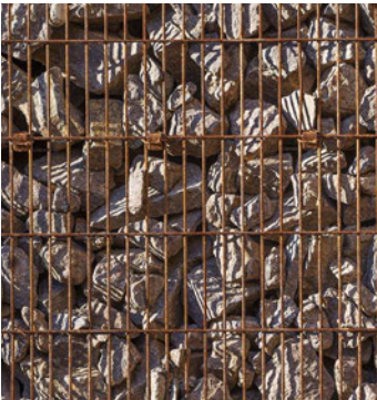
DWF Gabion Wall
