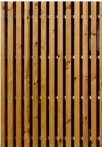
TMB2 Timber Battens - Vertical
